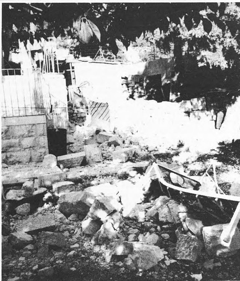
Partially demolished house belonging to West Bank Palestinian accused of resistance activity.
