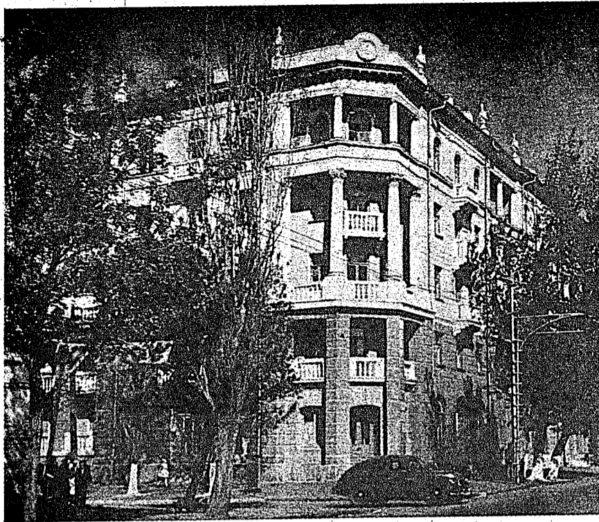
A newly-constructed workers' apartments house. The Plan envisages: 15,000,000 new flats and houses in the towns and 7,000,000 in the countryside.
