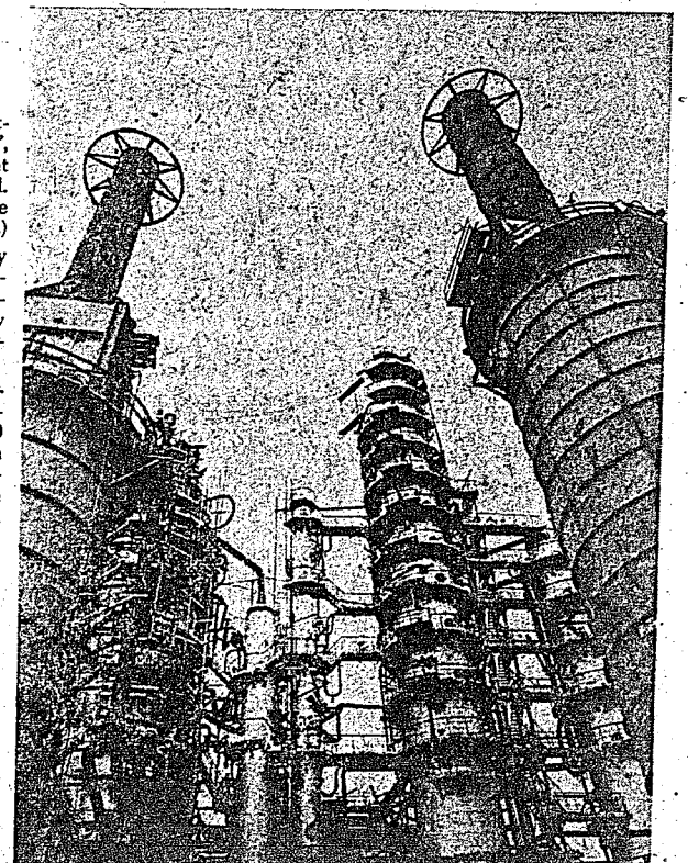
Oil Refinery at Plock
