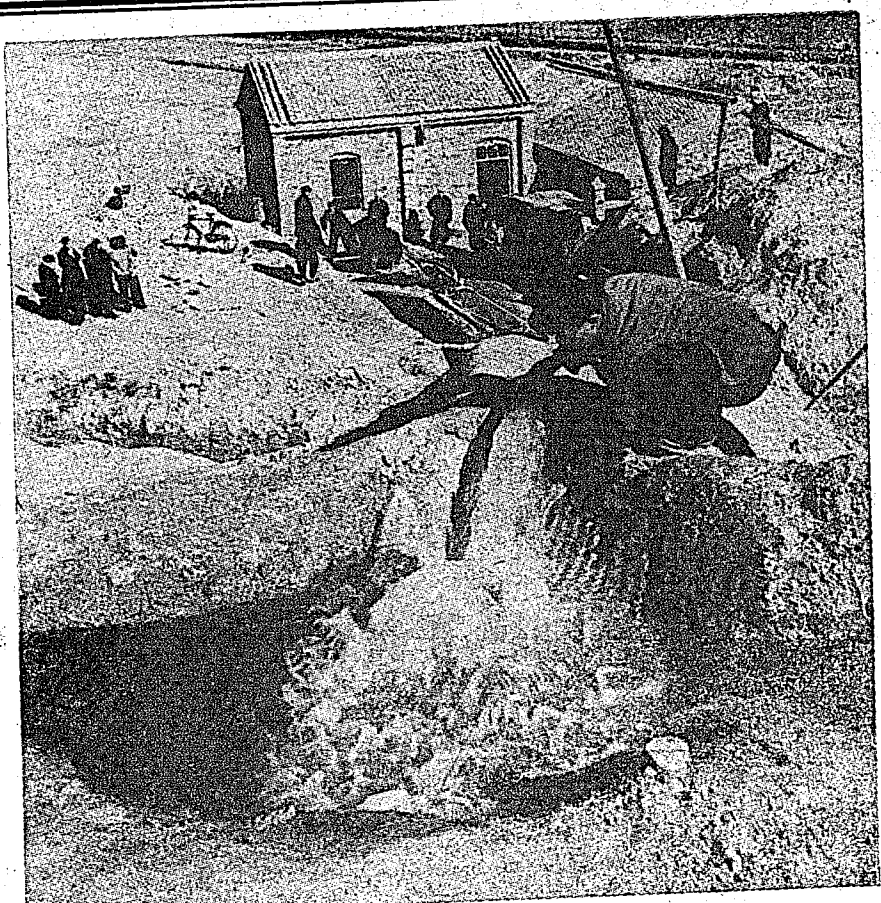
The electric power industry in China has also begun to walk on "two legs"—with big modern power plants and small ones operated by the masses of the people. Picture above shows a rural power station in Chinpi village in Shansi Province. The Hunng-nao County where this village is situated has already set up 62 such hydro-electric stations and power stations.—Photo: HUA KAI.
