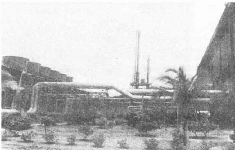
The Makban geothermal power plant.
