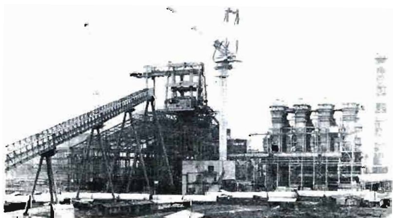
The 113-metre-high blast furnace under construction.
