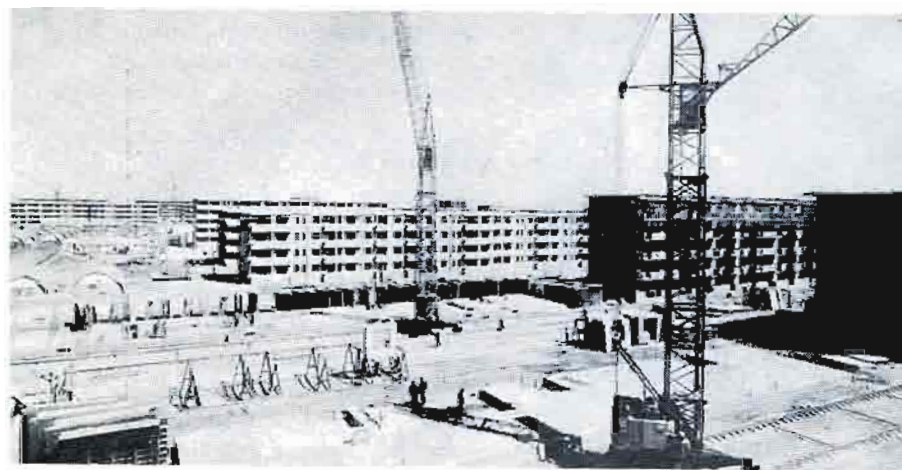
Part of the new Tangshan under construction.
