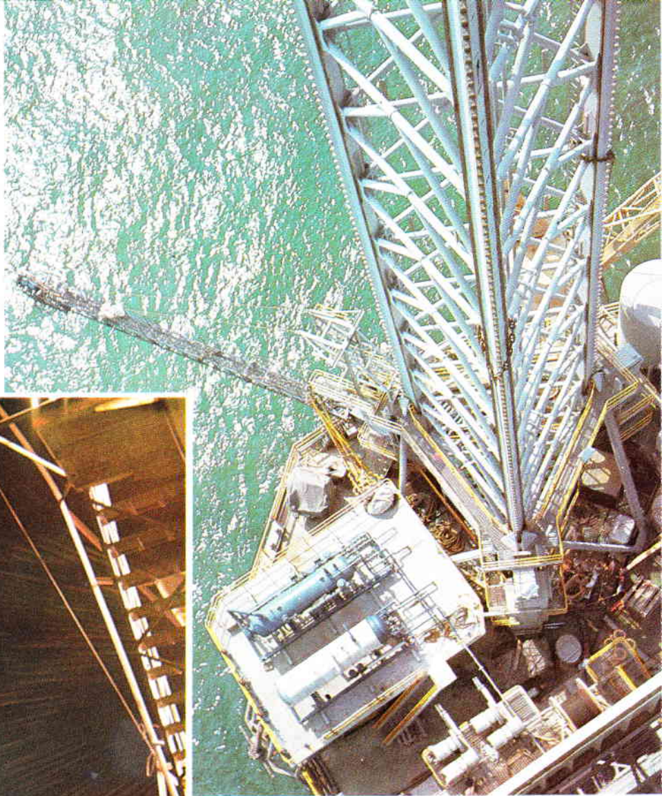
Three extendable steel legs automatically keep the platform 10 meters above sea level.
