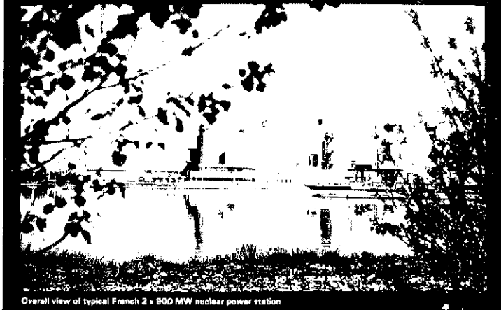
Overall view of typical French 2 x 900 MW nuclear power station
