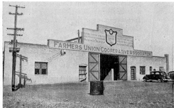
In the right wing of this building, Williston, North Dakota, the 1937 Cooperative Institute was held.
