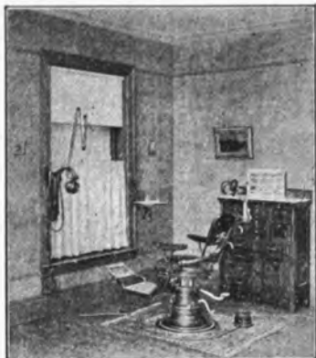
Showing the Folding Bracket Engine fastened to the wall, with the motor and arms as positioned when not in use.
