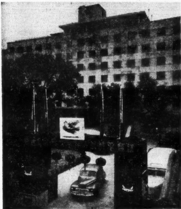
"NOTHING IS IMPOSSIBLE" to the Chinese, reported N. Y. building contractor Henry Willcox. Completion of the Peace Hotel (above), where the delegates stayed, was rushed in two months; the same work would take six here. Supervising engineer Yang praised the suggestions for solving critical problems made by the 900 men on the job. A week before delegates arrived, 100-ft. scaffolding surrounded the building; they found it furnished, immaculate, complete with elevators, curtains, linen and china and silverware marked with Picasso's dove of peace. Commented Willcox: "I have been putting up buildings for 40 years, and I am frankly stumped by the speed of this job."
