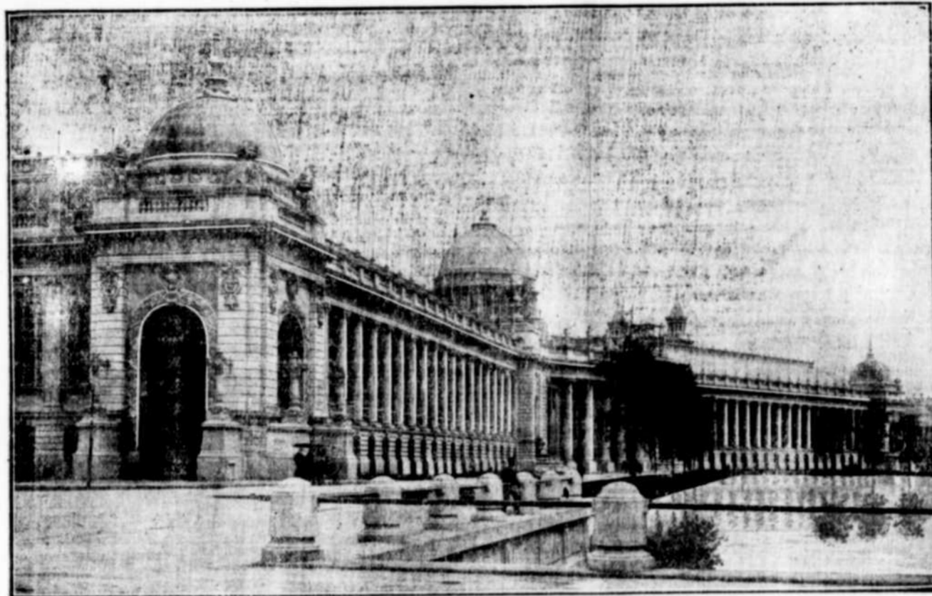
VARIED INDUSTRIES BUILDING AT E POSITION.
