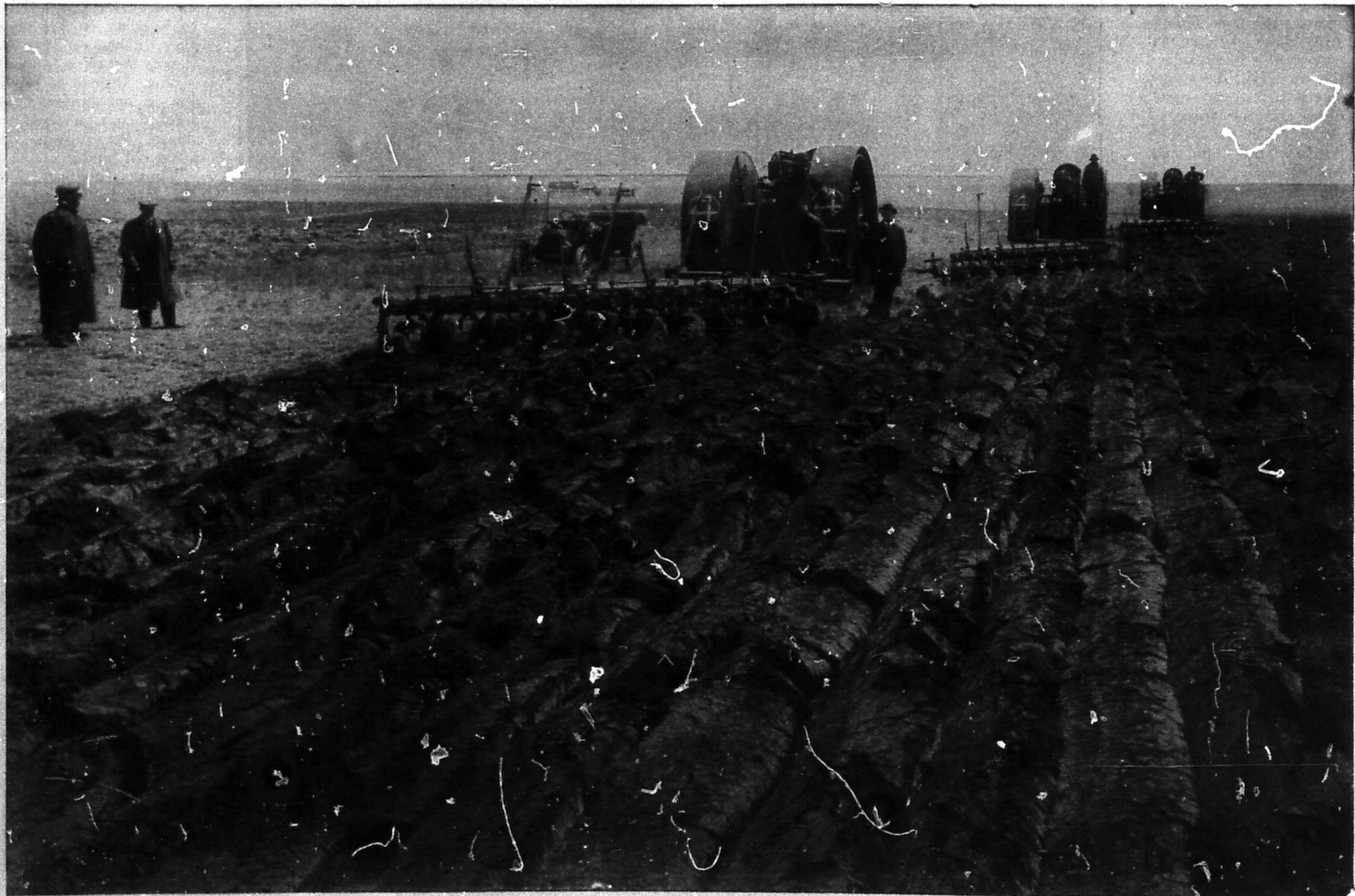
Battery of gas engines double-discing an enormous acreage
