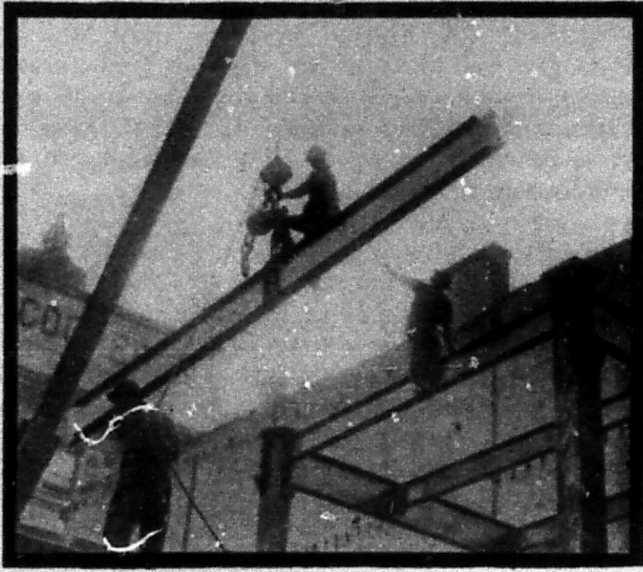
Fitting a girder into place
