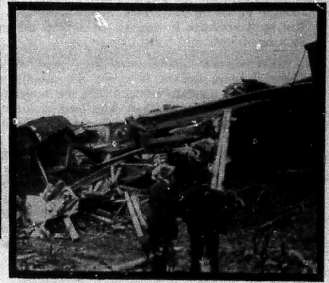
Wreck of the Twentieth Century Limited
