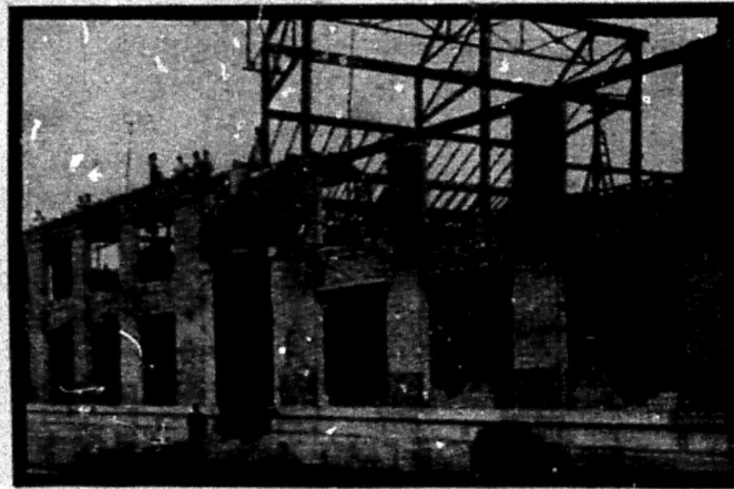
Shoe Factory Under Construction at Lillers
