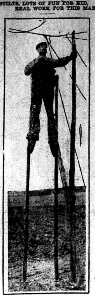
Here's a man who walks on stilts for a living. His stilts are about 16 feet long, and the wook blocks for his feet to rest on are twelve feet from the ground. He works in a big hop field. Hops, you know, grow very tall, on strings, just like vines. This man's job is to fasten up the strings, which are tied at the top to a line strung between high poles. The hop field where he works is in England.
