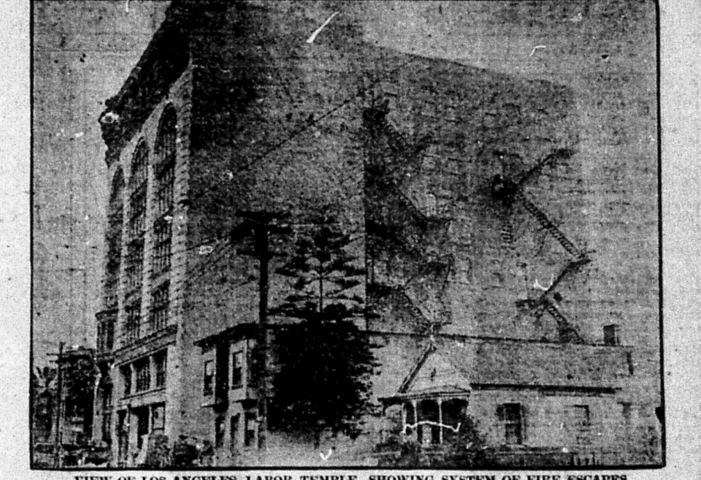
VIEW OF LOS ANGELES LABOR TEMPLE, SHOWING SYSTEM OF FIRE ESCAPES.
