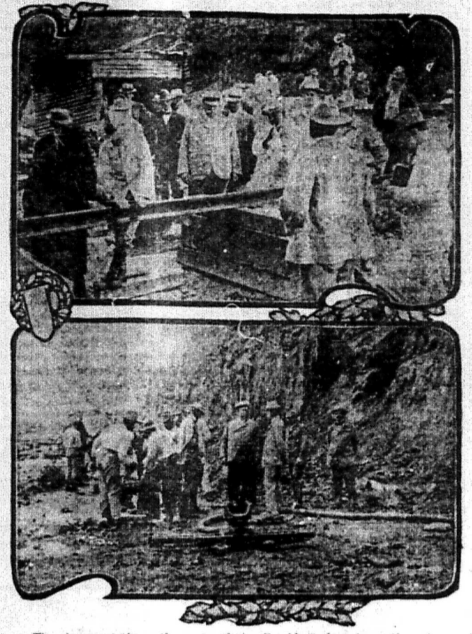
The above out shows the party of the President-elect inspecting the work at Panama.
