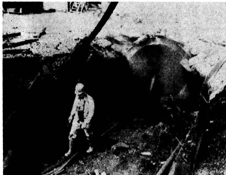
Damaged entrance to Borken mine after coal dust explosion killed 51 miners.
