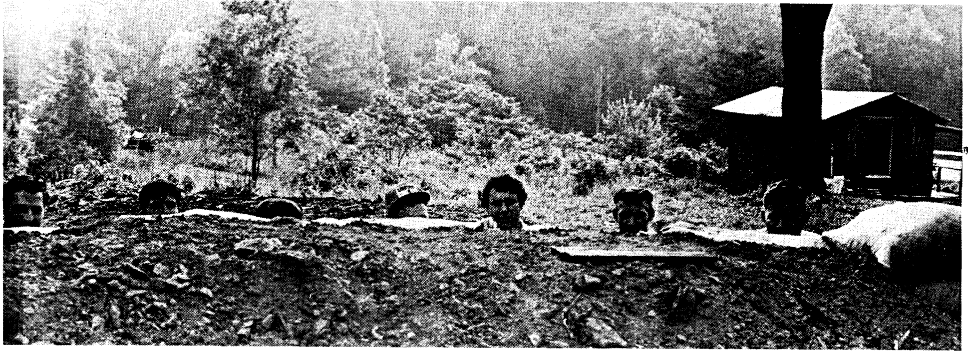
Stearns miners in trench outside union hall at Justus Mine.
