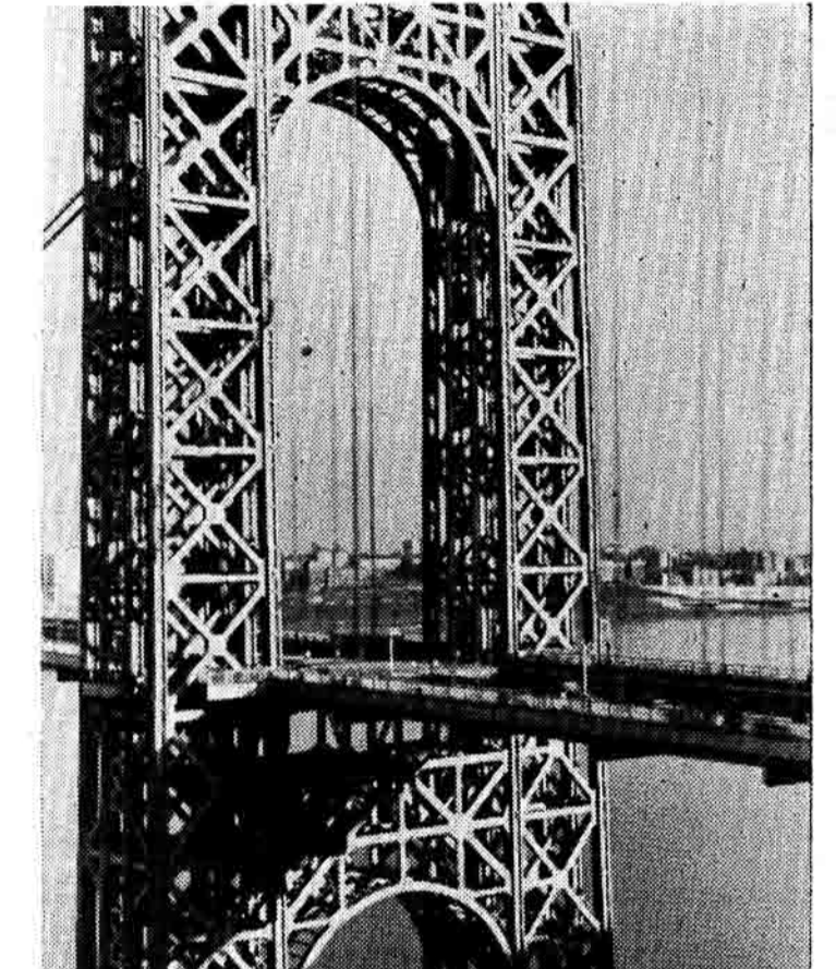
George Washington bridge. Patriotic New Yorkers consider it one of the world's most beautiful structures. To the Port Authority, the most beautiful feature seems to be the toll booth where motorists are stopped as if they were at the gates of a Middle Ages barony. Congressman Celler says tolls have paid for the bridge twice over.
