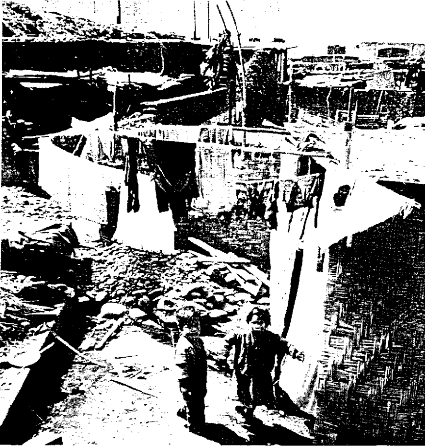
This picture was taken over five years ago of a shanty town in Lima. There was no water or sanitation, the dwellings of the shanty town gave little protection from the intense heat or chilling fog - even then it was a "fine breeding place for disease". The source of the photograph? One of the United Nations organisations.
