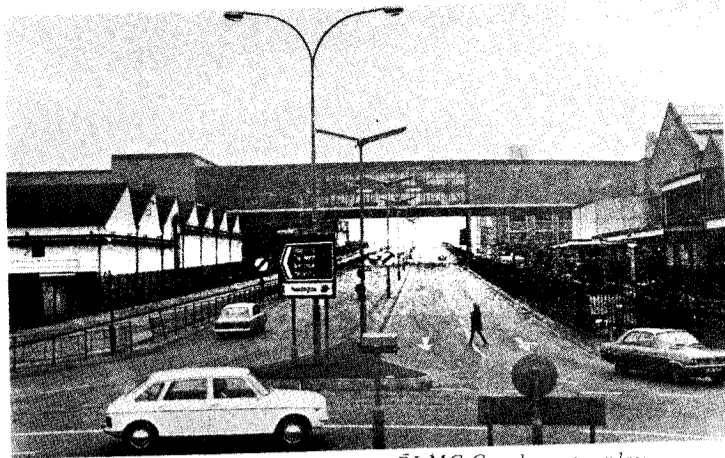
BLMC Cowley complex
