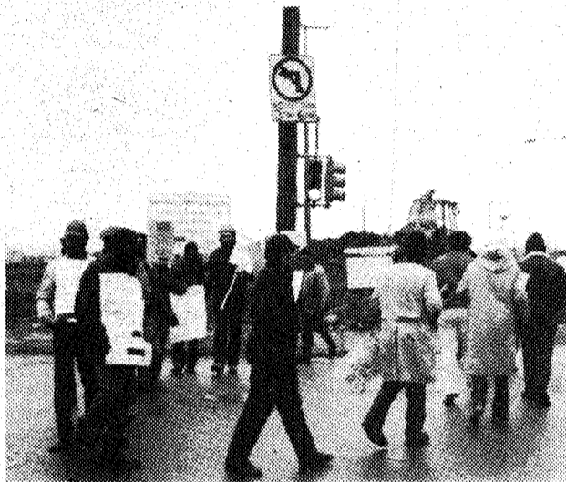
Pickets stop construction in Poletown.
