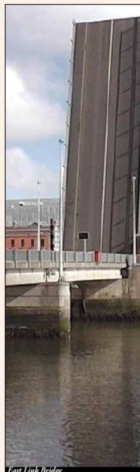
East Link Bridge
