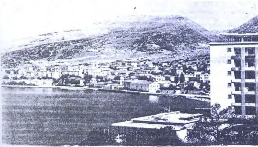
Workers' flats in Saranda. The Albanian State supplies materials and workers supply the voluntary labour to build homes for themselves and their comrades.
