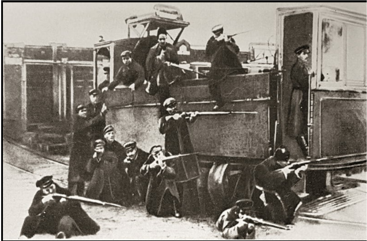
A reinforced tram platform used in the November fighting in Moscow's Zamoskvorechye District.
